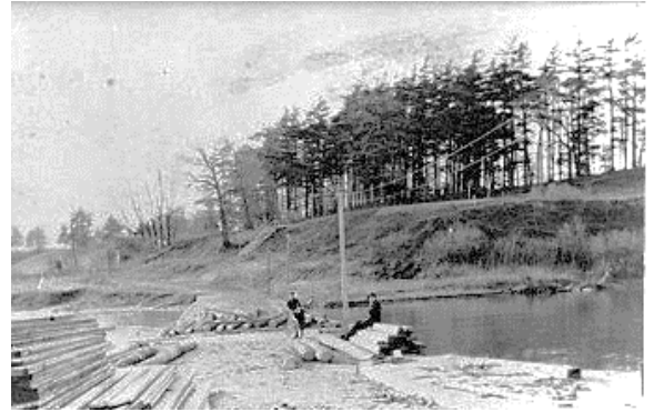
This photo is of the embankment at Brown's Wharf, Aldershot. The embankment at the bottom of Locust Street would have been similar.
