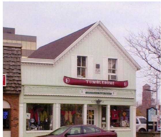
401 Brant Street, ca 2010 BHS Archives
